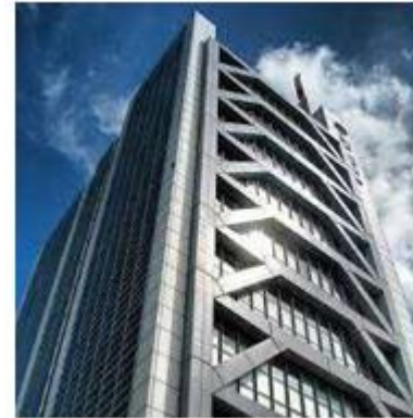
Fig2.6 Eccentric bracing
