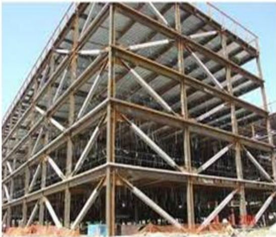
Fig 2.7 Buckling Restrained Brace
